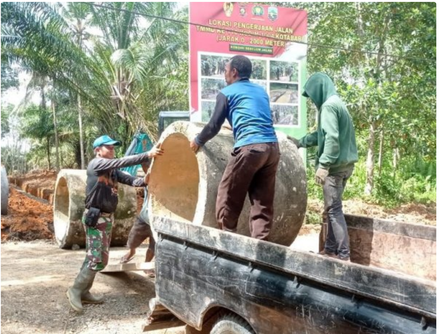
Cegah Genangan Air, Satgas TMMMD ke 116 Kodim 1004 Kotabaru Pasang Gorong - Gorong
